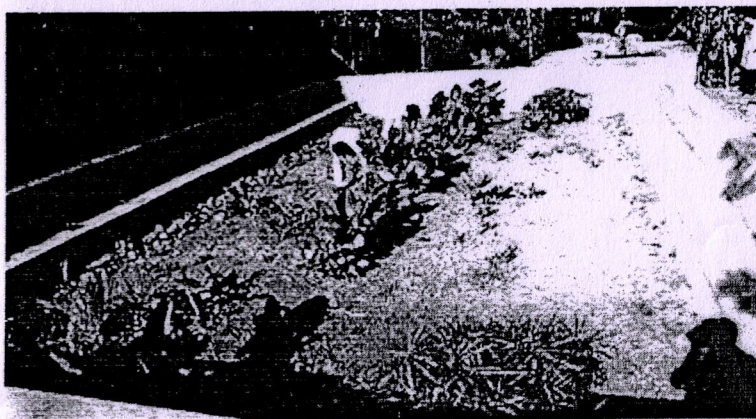
DEWAT Plant at Sane Guruji Hospital (Planted Gravel filter)
